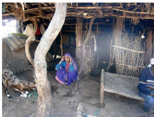
Goat shed constructed by Vair Singh, using locally available material, has been divided into 2 parts to avoid over-crowding.
